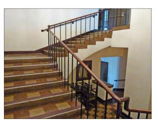
In 1980 Stairwell No. 3 was substantially modified to meet modern fire codes. Original openings were walled off with steel fire doors, no attempt was made to integrate this new work with the aesthetics of the original building. This stairwell was an important part of the ceremonial passage through the building and per the original design also functioned to bring light to the hallways on each floor that the stairwell serves. These modifications were
